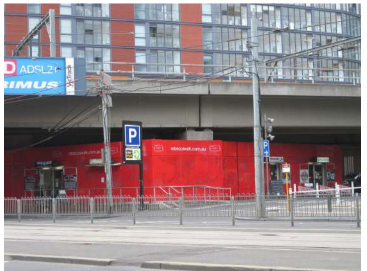
Melbourne's Rebecca Walk features pop-up retail under a rail viaduct. Credit: Mike Lydon
