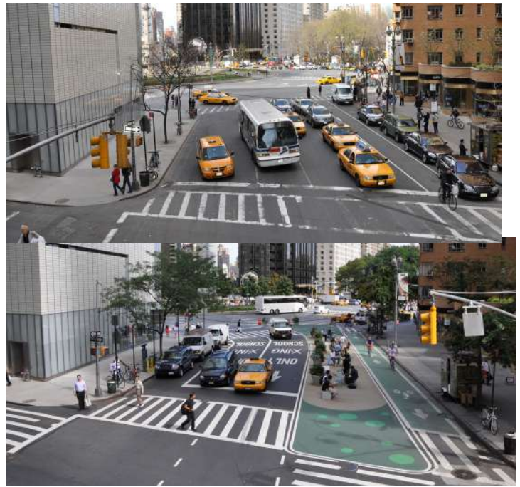
Broadway at Columbus Circle: Before and after. Credit: New York City Department of Transportation
