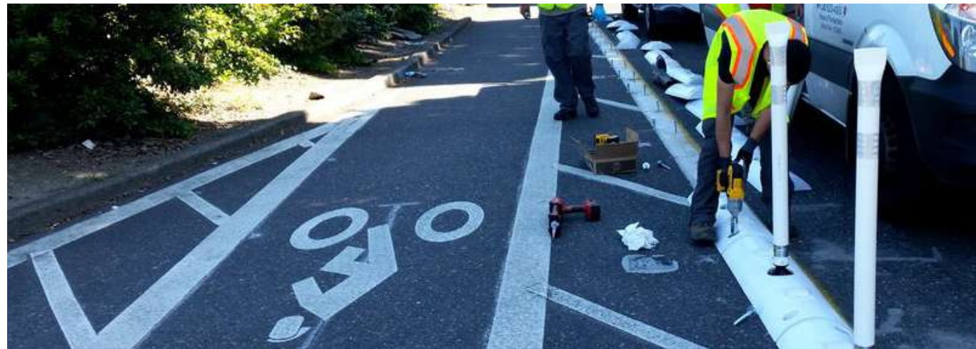
Top left: Flexible delineators proved ineffective at SW 13th Avenue and Clay Street (Jonathan Maus, Bike Portland); Top right: Raised lane separators provided a more robust barrier between people driving and people cycling (City of Portland Bureau of Transportation); Bottom: Raised lane separators are bolted into the asphalt (City of Portland Bureau of Transportation).
