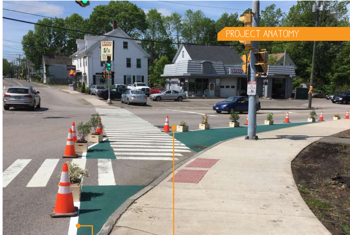
A generous curb extension reduces the turn radius and shortens the crossing distance by 20% (Street Plans).
