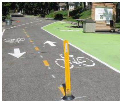
Flexible delineator - see page 28 - at the North Minneapolis Greenway pilot project (Carrie Christensen).
