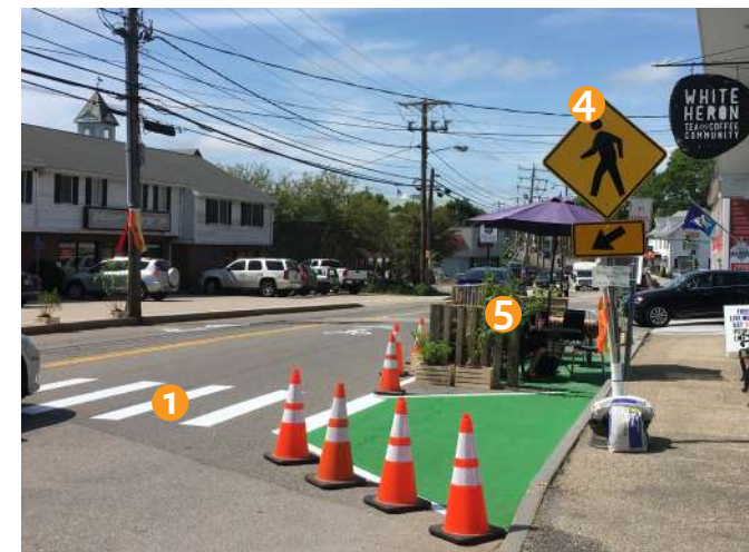
Above: A median refuge made out of straw wattle, hay bales, and flowers improve the walking (and rolling!) experience in Ponderay, ID (Street Plans). Below: A new crosswalk and curb extension improved the visibility of people walking along Portsmouth, NH’s Islington Street (Street Plans).
