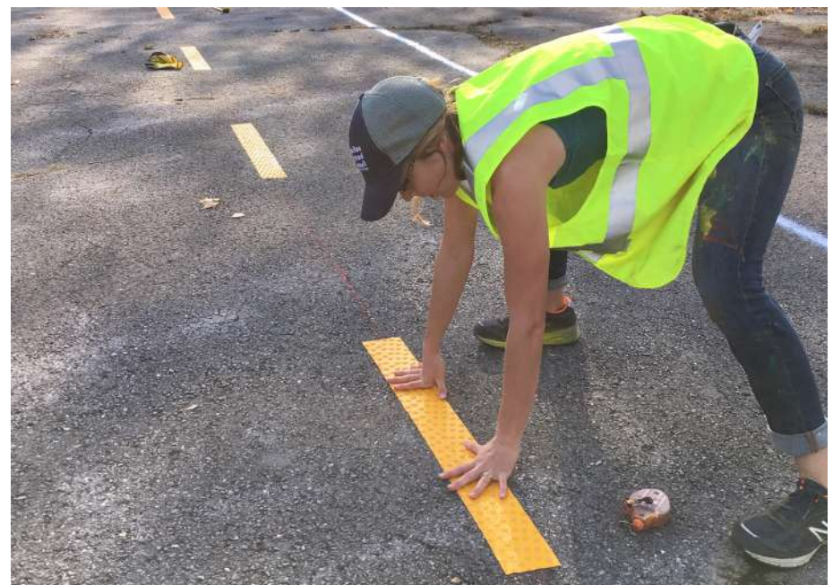
Contractor grade traffic tape is used to demarcate the center line of a monthlong protected bikeway project in Bella Vista, AR (Street Plans).
