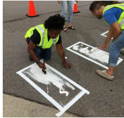
Left: Volunteers create a demonstration protected bikeway in Detroit using spray chalk (Team Better Block). Right: Volunteers use white duct tape and white tempera paint to create a new crosswalk along Detroit's Michigan Avenue (Street Plans).
