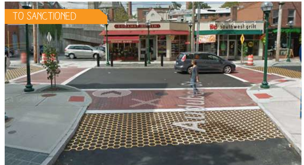
Above: An unsanctioned crosswalk highlighted a real need at the Whitney Avenue / Audobon Street Intersection (Thomas Macmillan, New Haven Independent). Below: Two years later the entire intersection was raised with new crossing treatments (Google).
