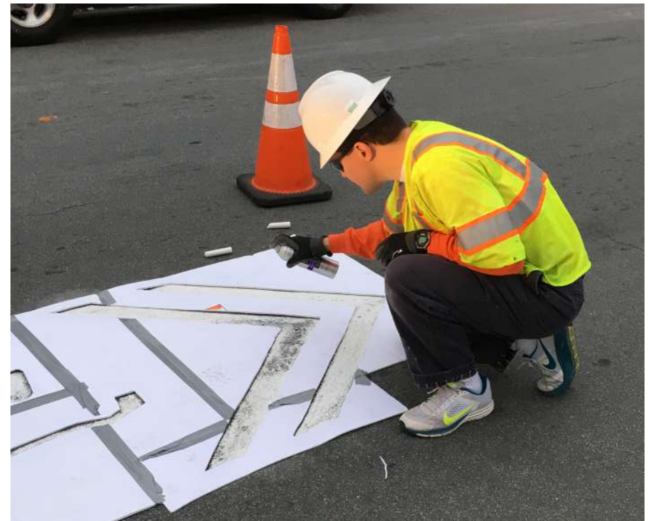
In San Jose, CA a volunteer applies hair spray to help set pavement marking created with sidewalk chalk. (Street Plans)
