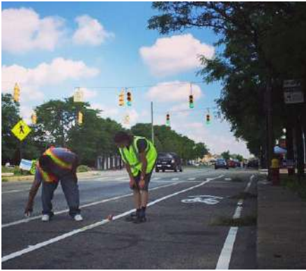
Left: Volunteers create a demonstration protected bikeway in Detroit using spray chalk (Team Better Block). Right: Volunteers use white duct tape and white tempera paint to create a new crosswalk along Detroit's Michigan Avenue (Street Plans).
