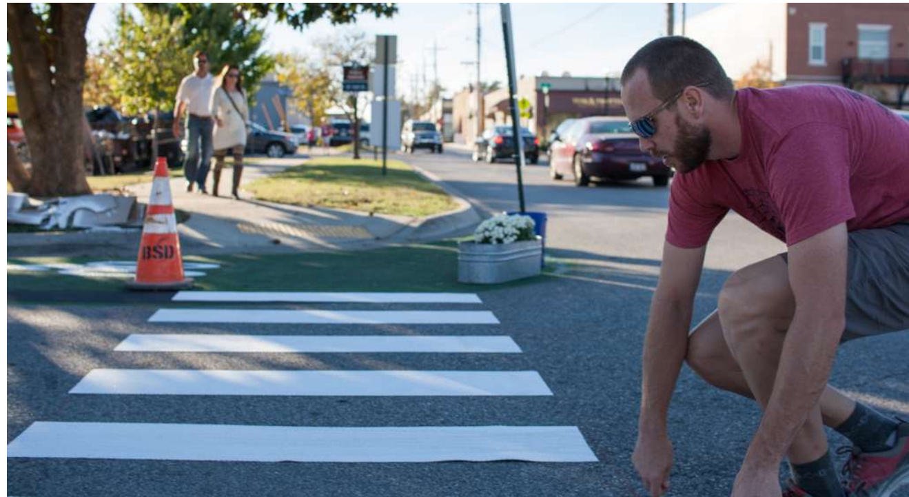
Above: Refreshing a faded crosswalk in Ponderay, ID (Strong Towns). Below: 12 in. wide strips of traffic tape and green spray chalk are used to create a crosswalk and traffic diverter along SE A Street in Bentonville, AR (Megan Sebeck).
