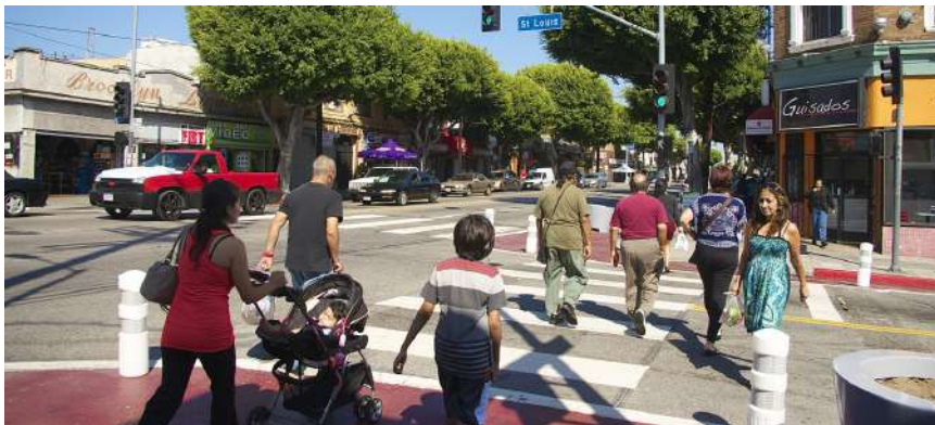
As part of the Vision Zero initiative, LADOT uses simple materials like striping, k-71 delineators (see page 31), and surface colorization (see 53 - 57) as an interim measure to tighten intersections, slowing turning vehicles and improving safety for people walking (LADOT/Jim Simmons).
