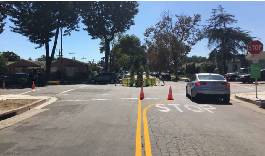
Foil-backed traffic tape is available in multiple colors, including yellow (seen here), which can be used for center line striping. Volunteers installed a very short-term splitter island with cones and yellow traffic tape to encourage people driving to navigate around a temporary mini-roundabout at the center of this Long Beach, CA intersection (Street Plans).
